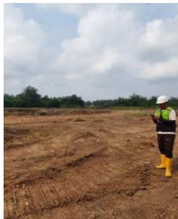
Use of PPE for employees
